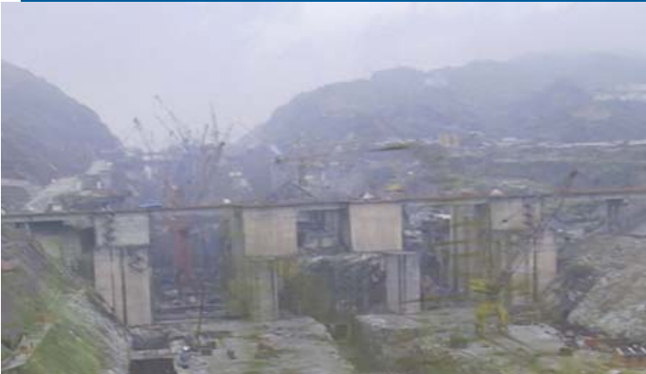
Foggy morning view of the Three Gorges Dam Project.
